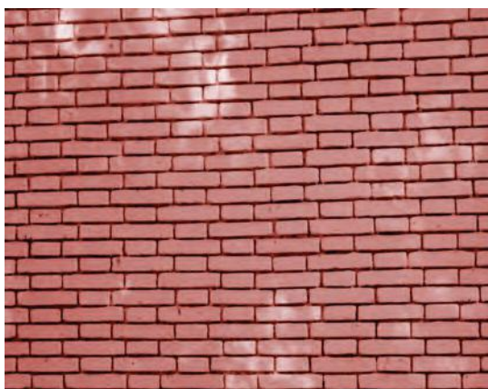
(a) Brick wall
