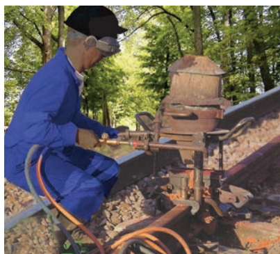
Figure 3.11 Thermit process for joining railway tracks
