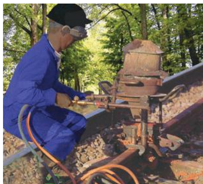
Figure 3.11 Thermit process for joining railway tracks
