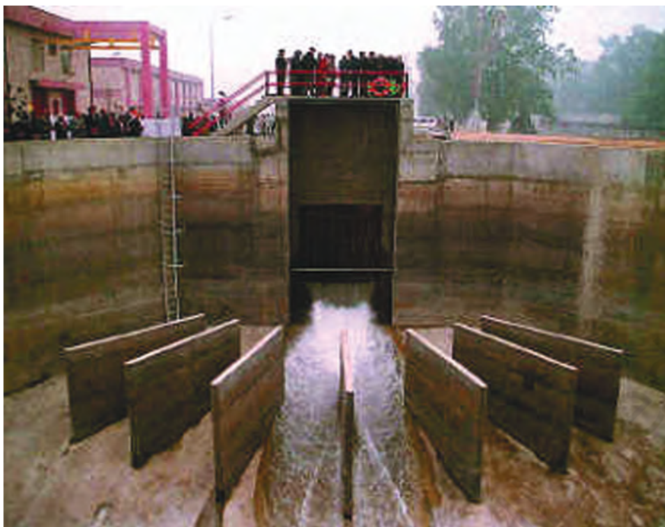
Fig. 18.10 : Water treatment plant
